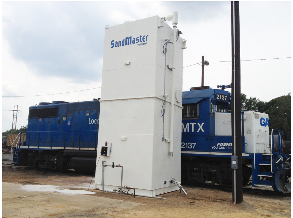
Pneumatic sand-filling systems, like Cyclonaire's SandMaster, deliver traction sand directly to the locomotive sandbox.
